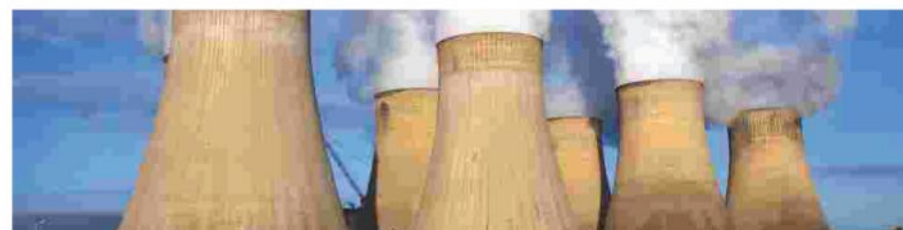
Power Generation Industry
